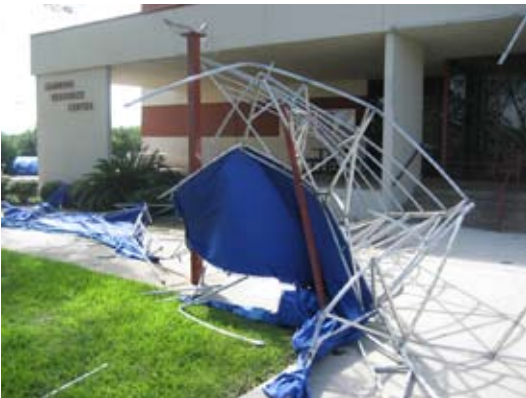
Damage inside and out at the LRC (left & below).
